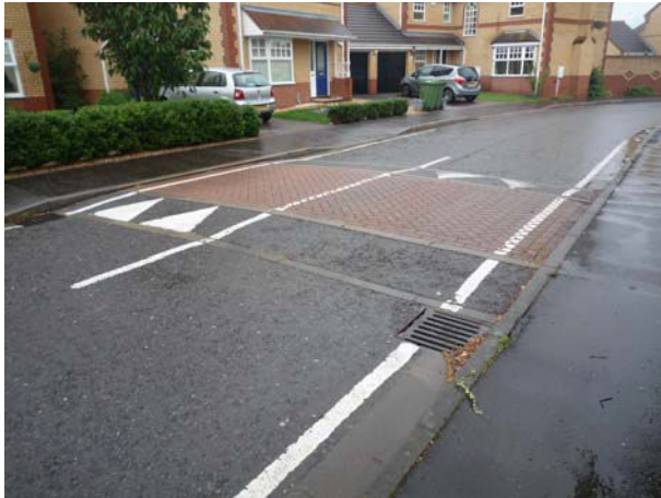
Raised carriage way makes a good crossing point but not flush with kerb and no blister warning
