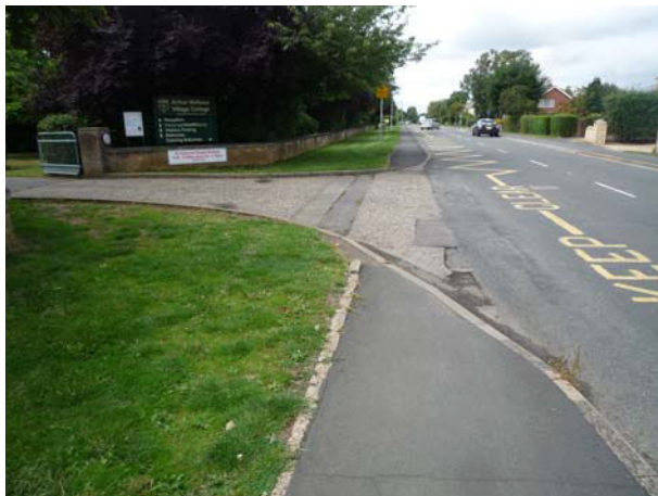
School entrance with no tactile warning
